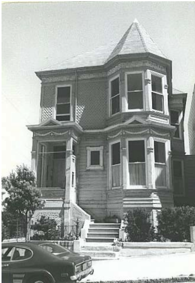
Figure 5. 722 Steiner Street, ca. 1976. In this photo, the portico has been closed in, and the exterior appears similar to how it looks today. The gate spanning the walkway to the south appears to be constructed of horizontal wood siding. (Photograph from San Francisco Planning Department, April 2015.)
