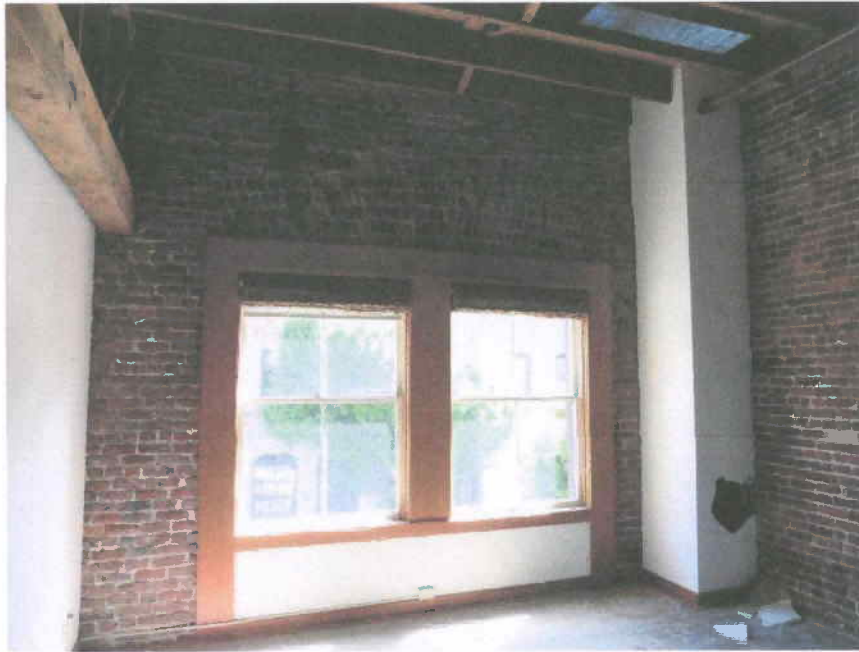
Interior of Montgomery Street 2 nd Floor windows
