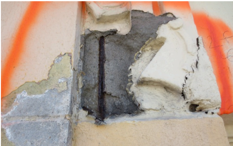
Figure 19. Exposed reinforcing bar at the twelfth floor along the north elevation. (Photograph provided by RLJC, April 2015.)
