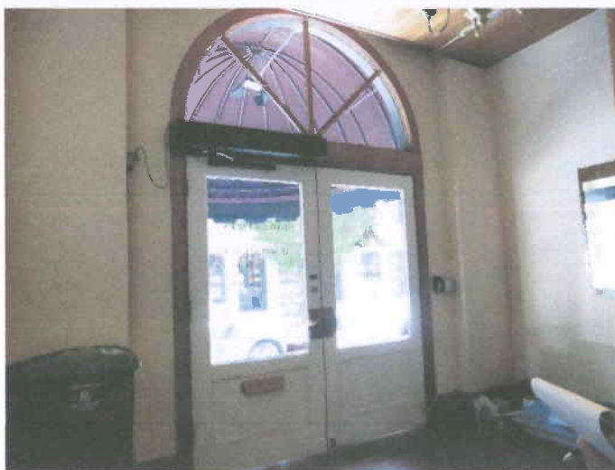
Interior of Montgomery Street entrance
