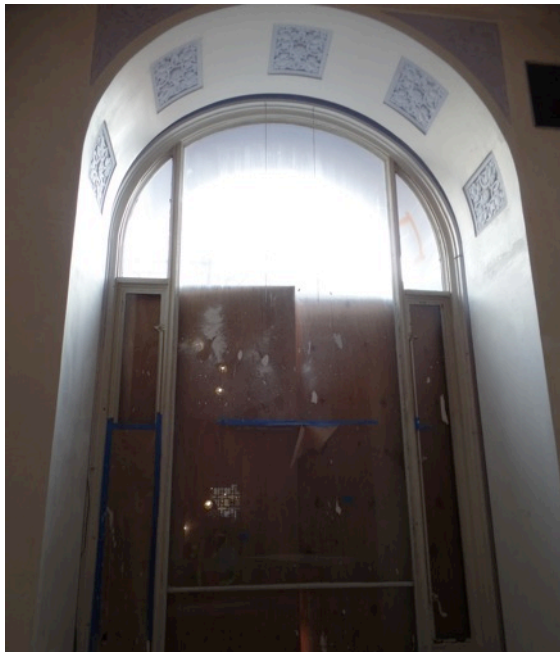
Figure 11. Overview of fixed and casement assembly at ground floor. The exterior is obscured. (Photograph by Garavaglia Architecture, Inc., April 2015.)
