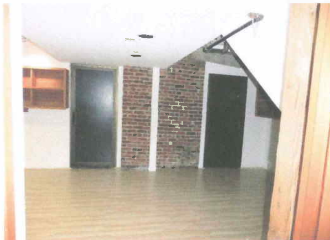
Basement with drop ceiling
