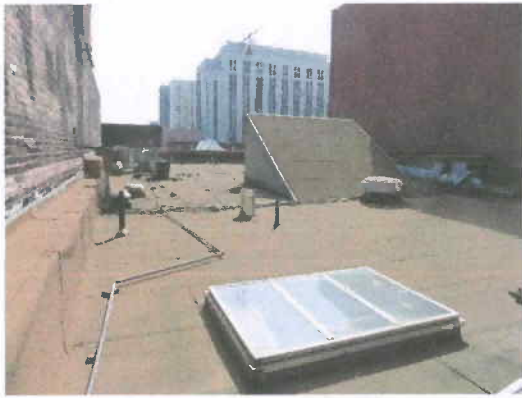
Roof overall, looking east
