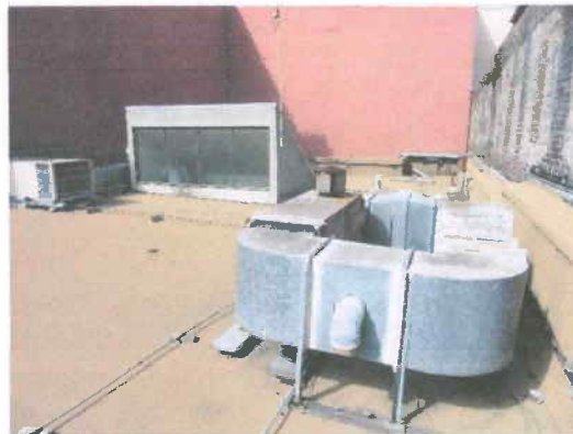
Roof, looking southwest
