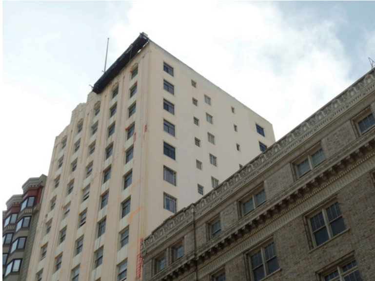
Figure 12. Overview of north and east elevations. (Photograph by Garavaglia Architecture, Inc., April 2015.)
