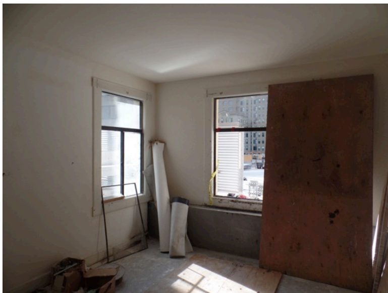
Figure 13. View of aluminum windows at off-street elevations. (Photograph by Garavaglia Architecture, Inc., April 2015.)
