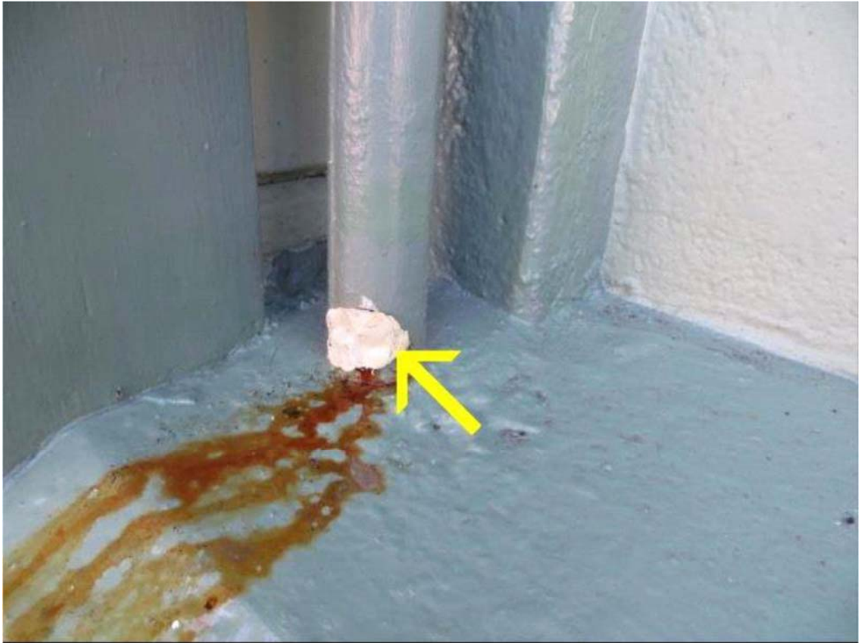
Corroded downspout
