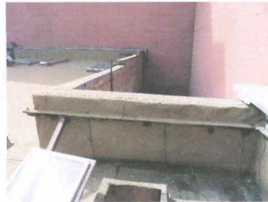
Roof and rear courtyard parapet
