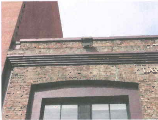
Montgomery Street Cornice Detail
