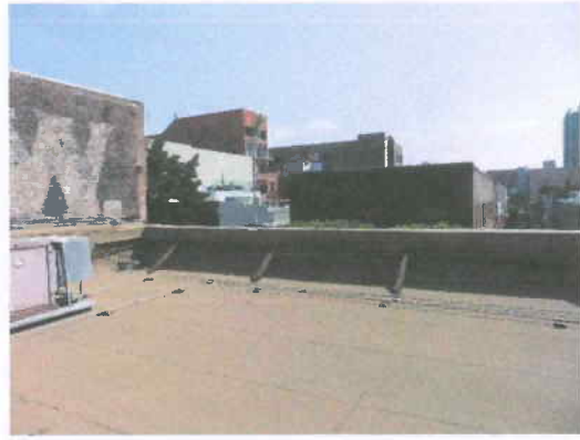
Roof with parapet braces
