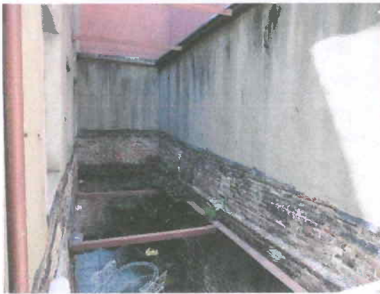
Rear Courtyard with bracing
