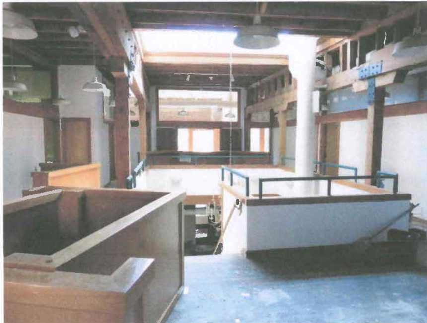
Overall of 2 nd Floor interior space, looking east
