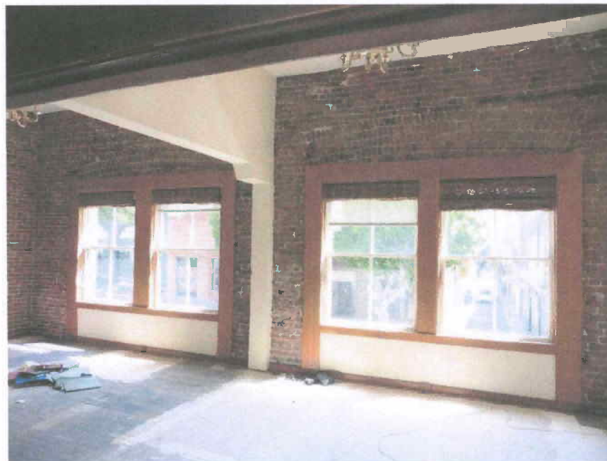
Interior of 2 nd Floor Montgomery Street windows
