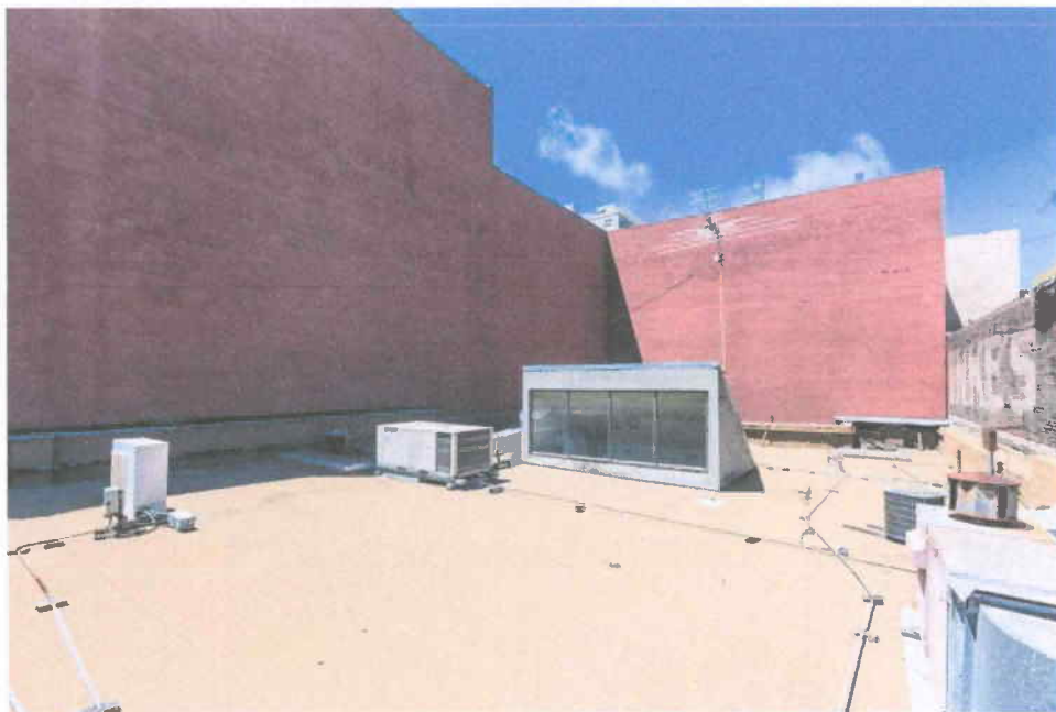
Roof Overall, looking west
