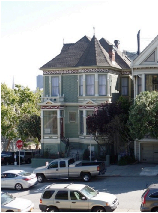
Figure 8. Overall view of west (Steiner Street) elevation. (Photograph by Garavaglia Architecture, Inc., April 2015.)
