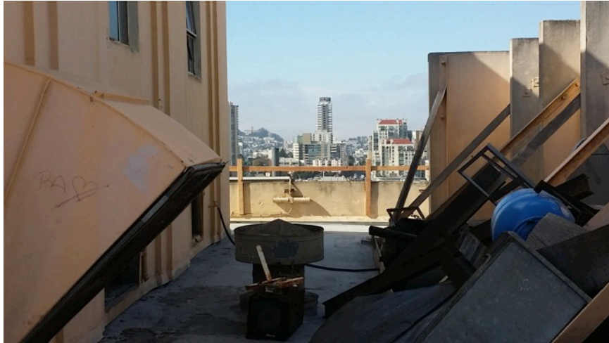
Figure 14. Overview of main roof level, showing mechanical equipment. (Photograph provided by RLJC, April 2015.)
