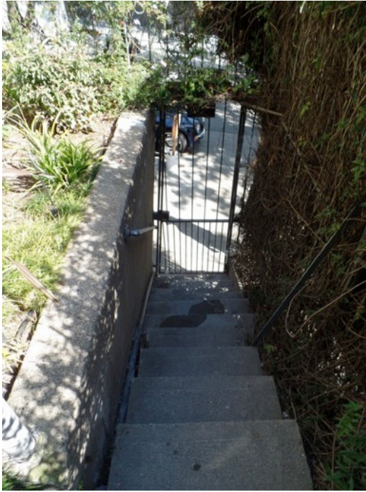
Figure 12. View of entrance gate and stairs to rear (east) elevation. (Photograph by Garavaglia Architecture, Inc., April 2015.)
